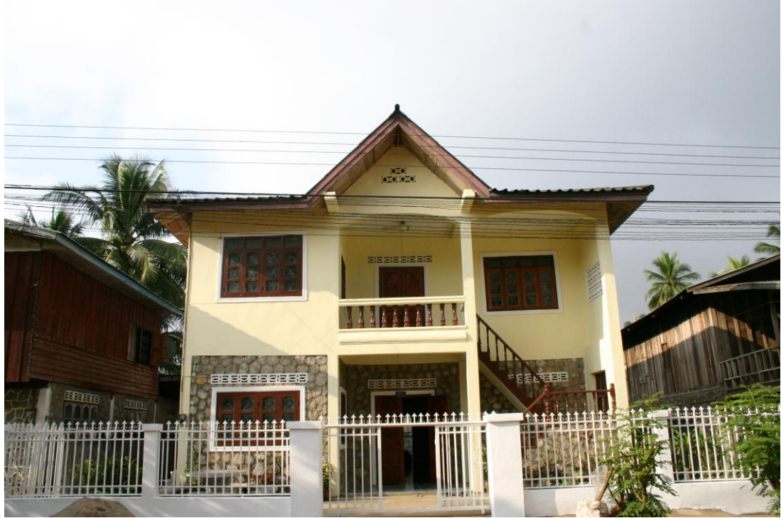
Figure 4: Grandma's newly remodeled house. (Luang Prabang, Laos, June 20, 1999)
